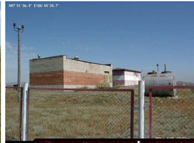
F. Hatch and tank
